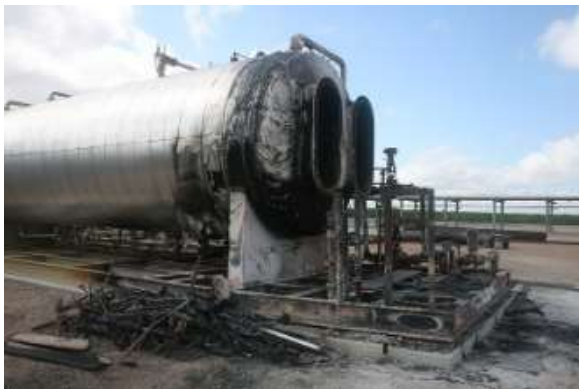
Figure 2: A damage to the burner end of a heater treater
